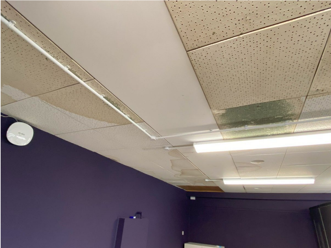
Sport and Media – Room 004 – mould and water staining from recent water ingress presents health and safety hazards
