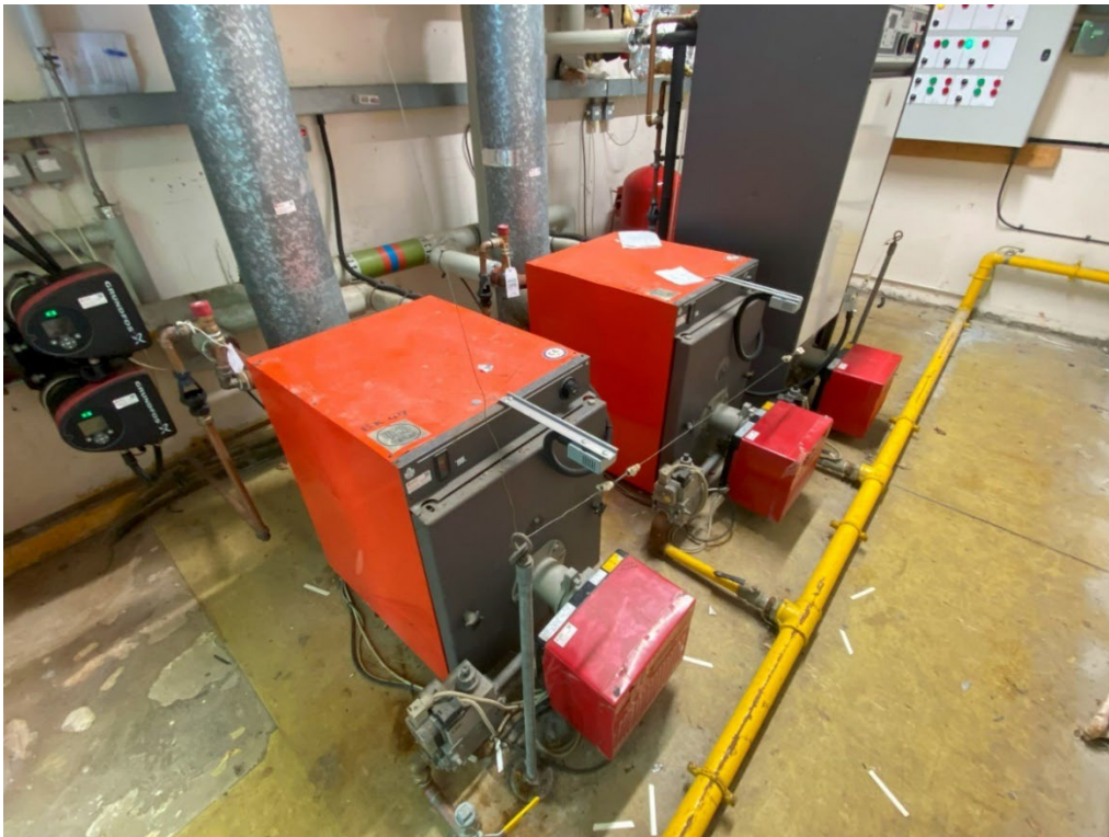
School of Art – Ground floor – two gas fired boilers and external burners require replacement being beyond their economic life
