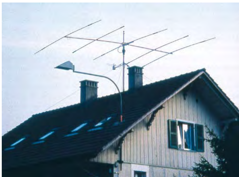
Amateur radio aerials can take very different forms. The one shown here is a Yagi roof aerial.
