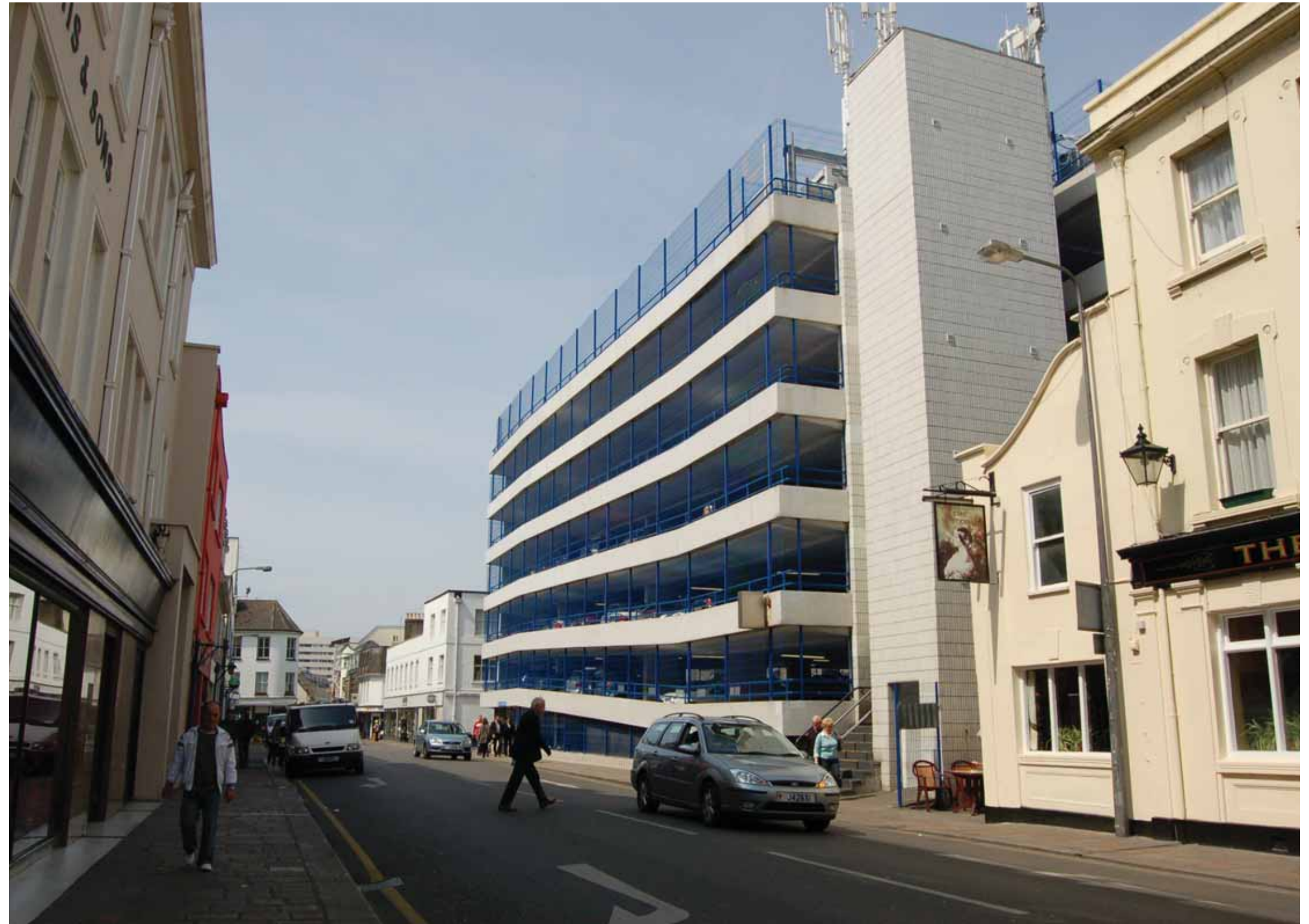
The existing Minden Place car park
