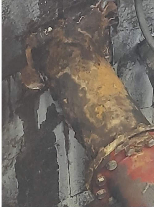
Photo B1.9.5 : Pontac connection to rising main
