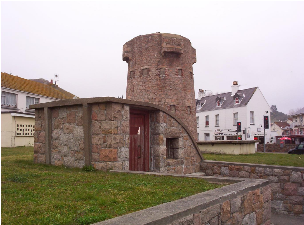
Photo B1.1.1 : First Tower above ground structure
