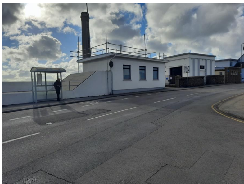
Photo B1.2.1 : Baudrette Brook (left) and Le Dicq (right) Pumping Stations
