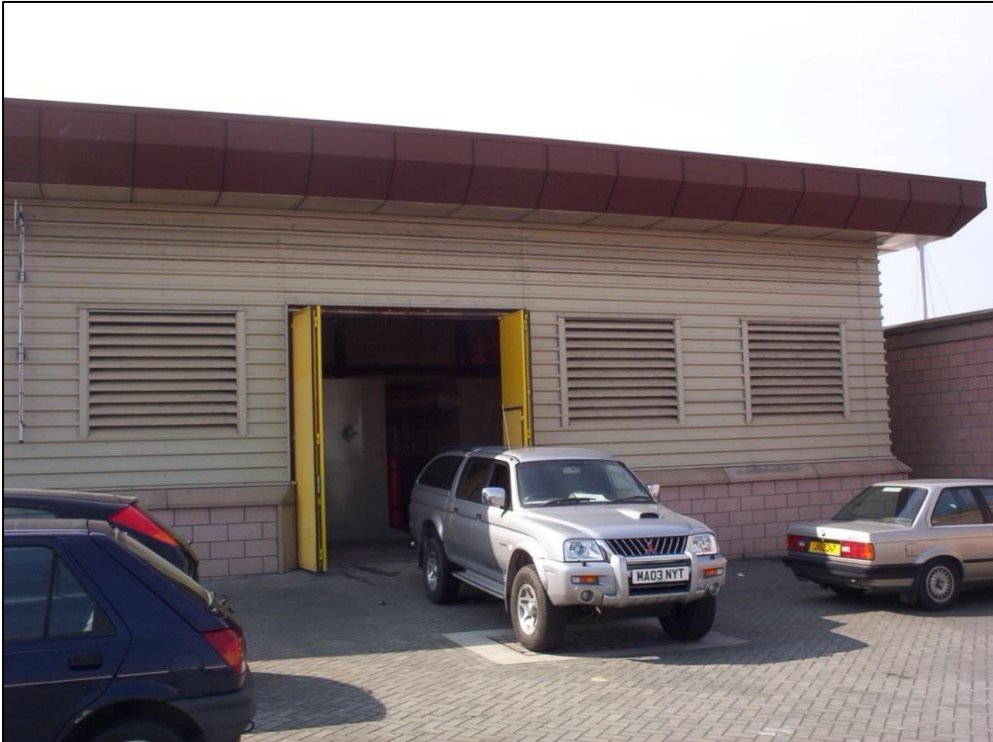
Photo J3.1 : West of Albert Pumping Station
