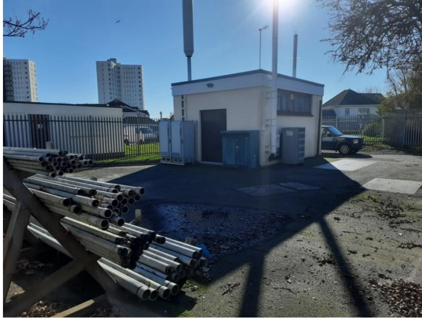
Photo B1.5.1 : Maupertuis pumping station above ground structure
