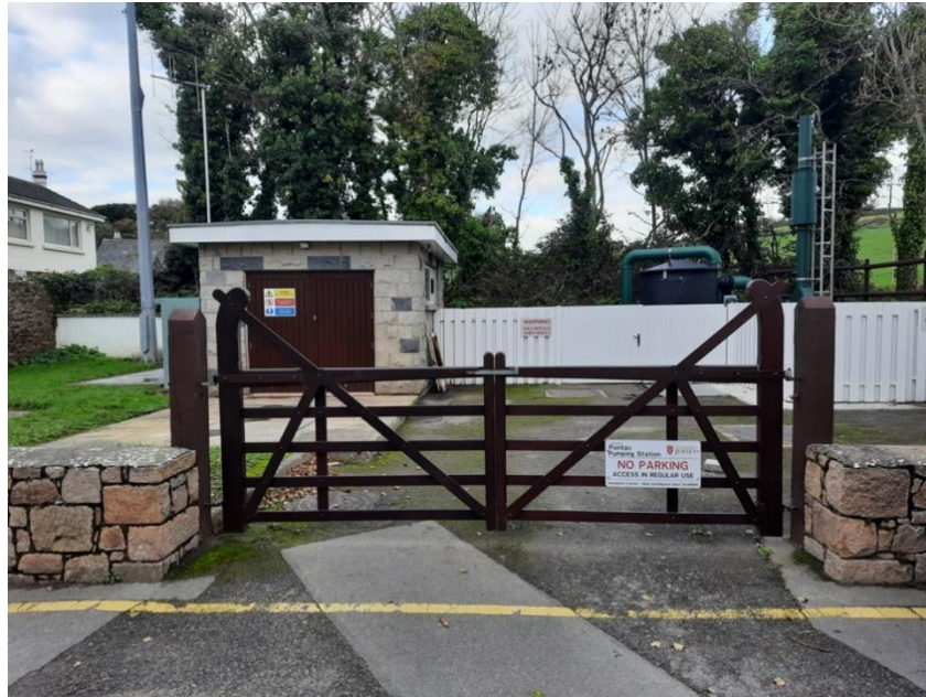
Photo B1.9.1 : Pontac above ground structure
