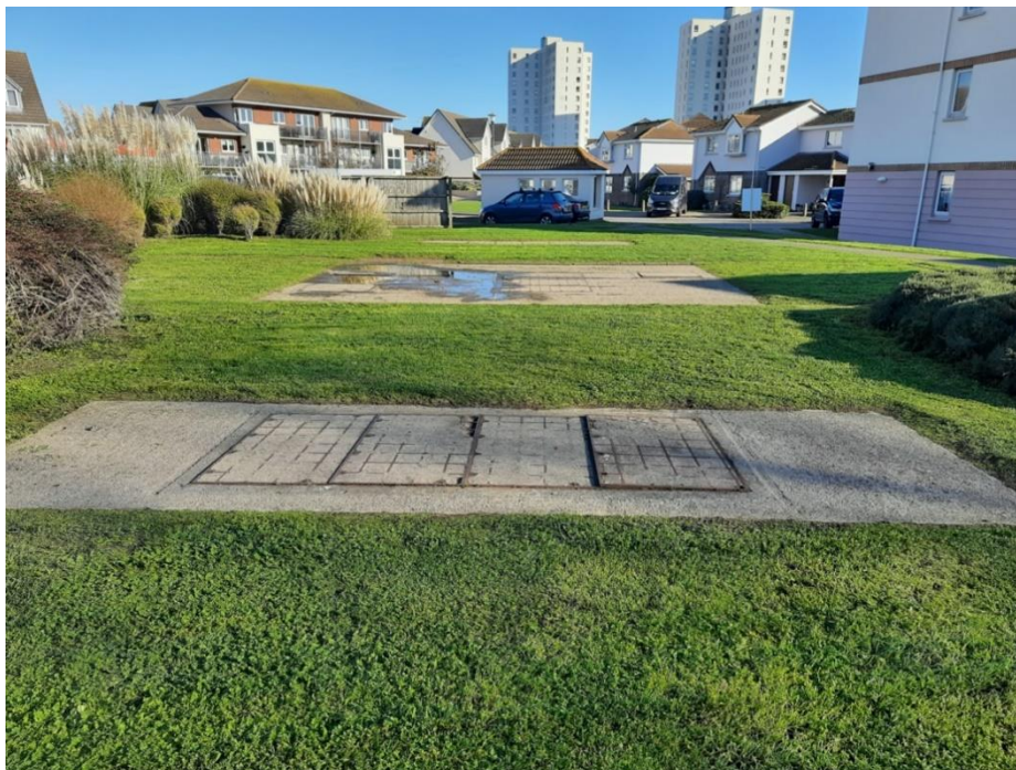
Photo B1.5.2 : Maupertuis Overflow pumping station
