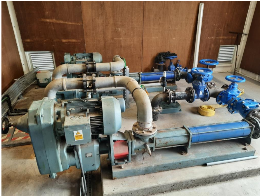
Photo J1.2 : Progressive cavity pump installation at La Route Du Port
