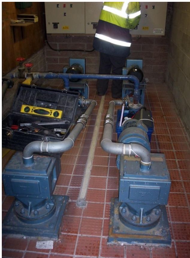
Photo E4 : La Collette Power Station PS Pump installation
