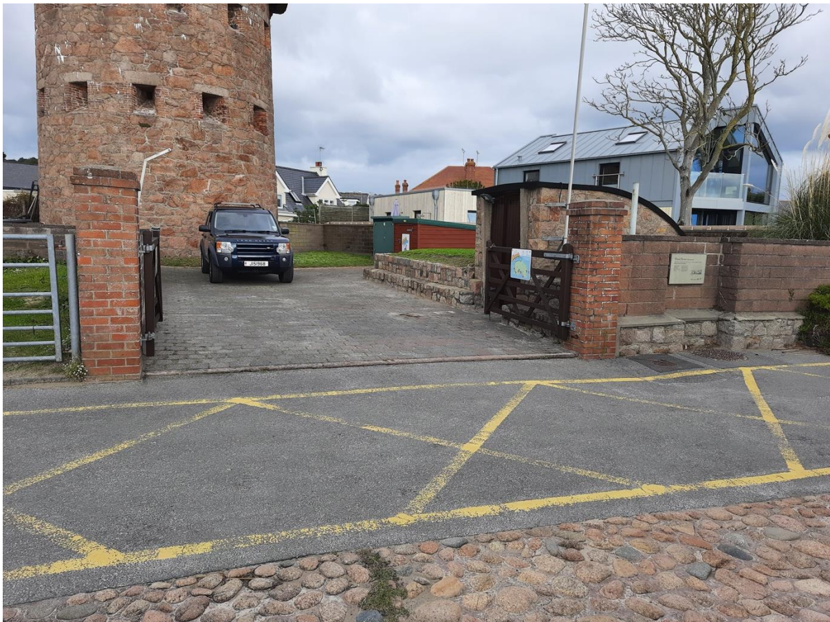
Photo B1.3.1 : Beaumont pumping station above ground structures
