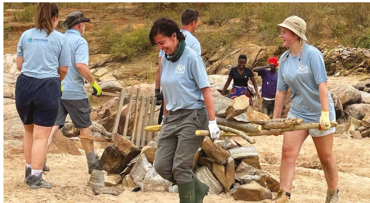
Volunteers building a sand dam in Kenya in June 2022
