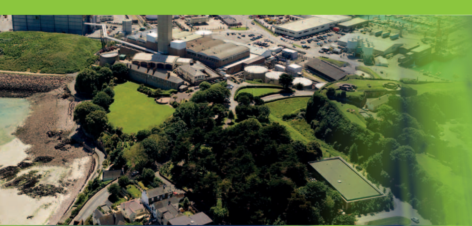
South Hill Switching Station
