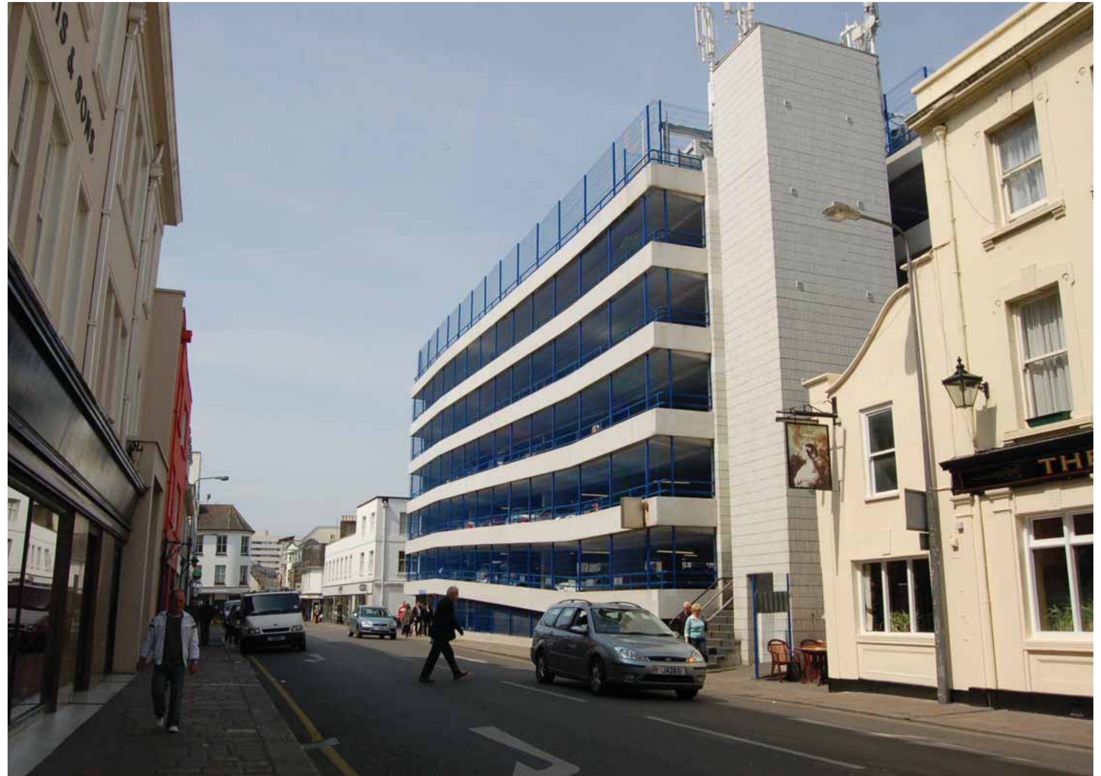
The existing Minden Place car park
