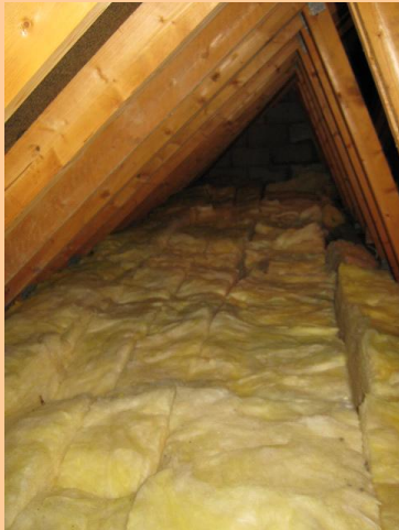
A freshly insulated section of loft in St Saviour.
