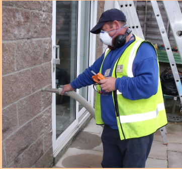
Cavity wall insulation being carried out in St Brelade.
