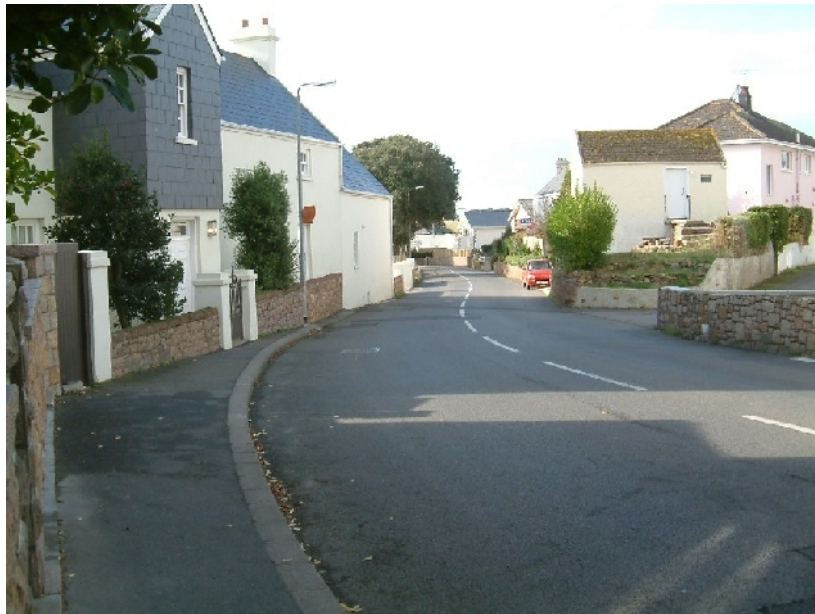
Plate 4: View of existing carriageway halfway between Pontac Slipway and Le Hocq.
