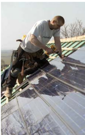
A building-integrated roof tile PV system and a conventional roof-mounted PV array. Source: XCO 2
