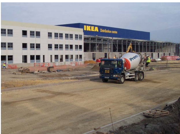
Ground source heat pump at IKEA's distribution centre, Peterborough. Source: EarthEnergy Ltd
