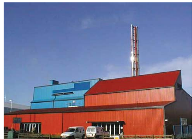
CHP plant serving Southampton's community heating network. Source: Southampton City Council
