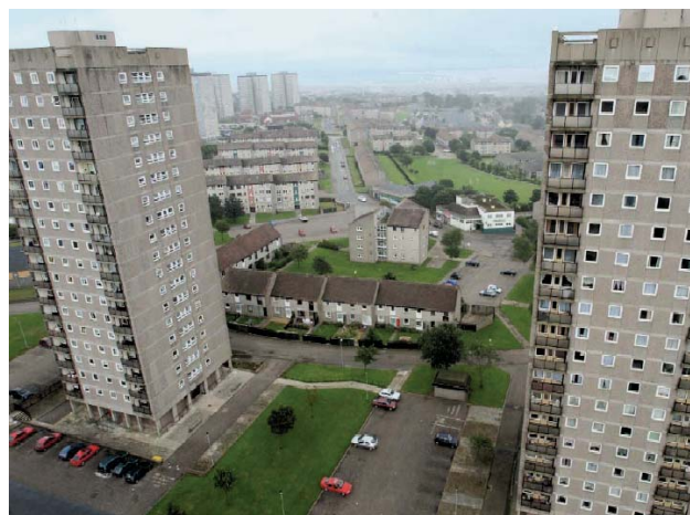
CHP installed as part of an affordable warmth programme, Aberdeen. Source: EST
