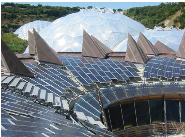
Solar PV array replaces traditional roof materials. Source: Solarcentury
