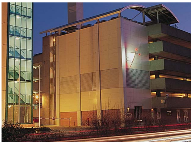
CHP, Woking. Source: Woking Borough Council
