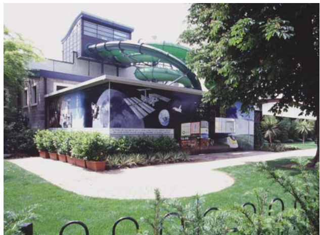
Fuel cell powered swimming complex operated by Thamesway Energy Ltd. Source: Woking Borough Council
