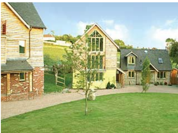
Homes in Shropshire built to high environmental standards. Source: Living Villages
