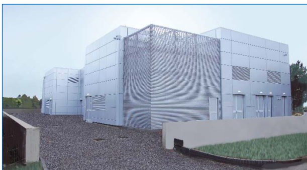
The new Western Primary sub-station
