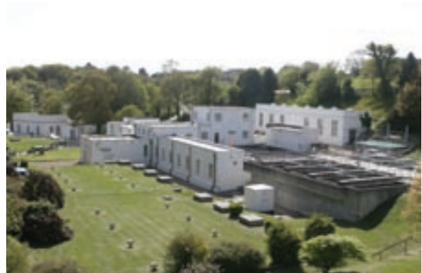
Handois Treatment Works
