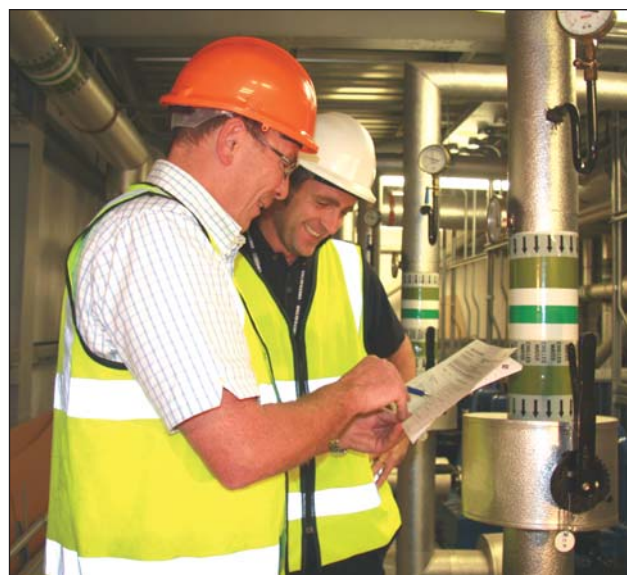
André de St George (Senior Health, Safety and Environmental Engineer) carries out a regular site inspection with Chris Young (JEBS)
