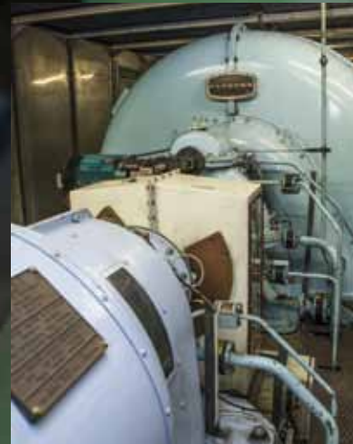
Main picture: Gauges on Sulzers' sea water cooling system.
