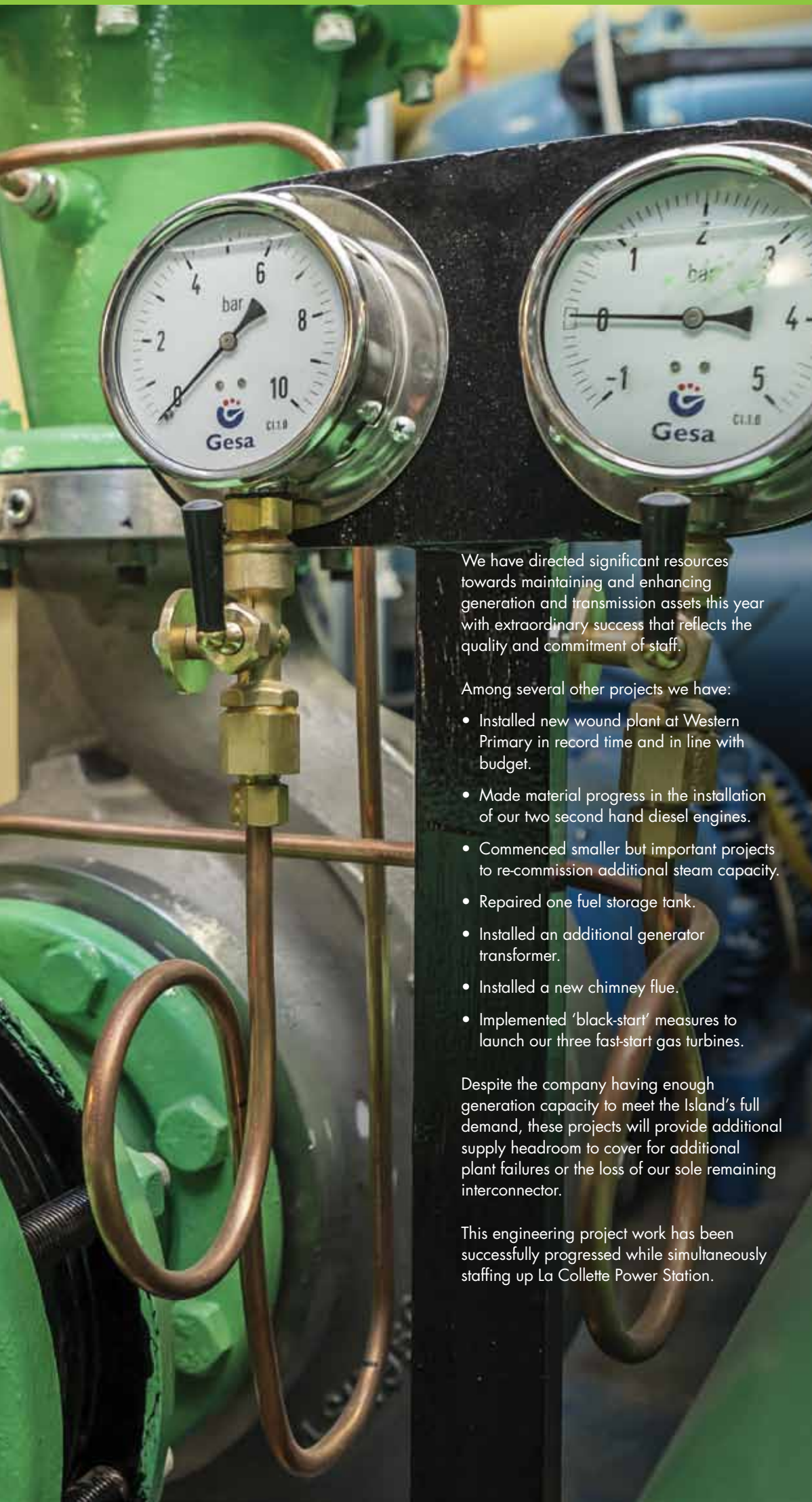
Main picture: Gauges on Sulzers' sea water cooling system.
