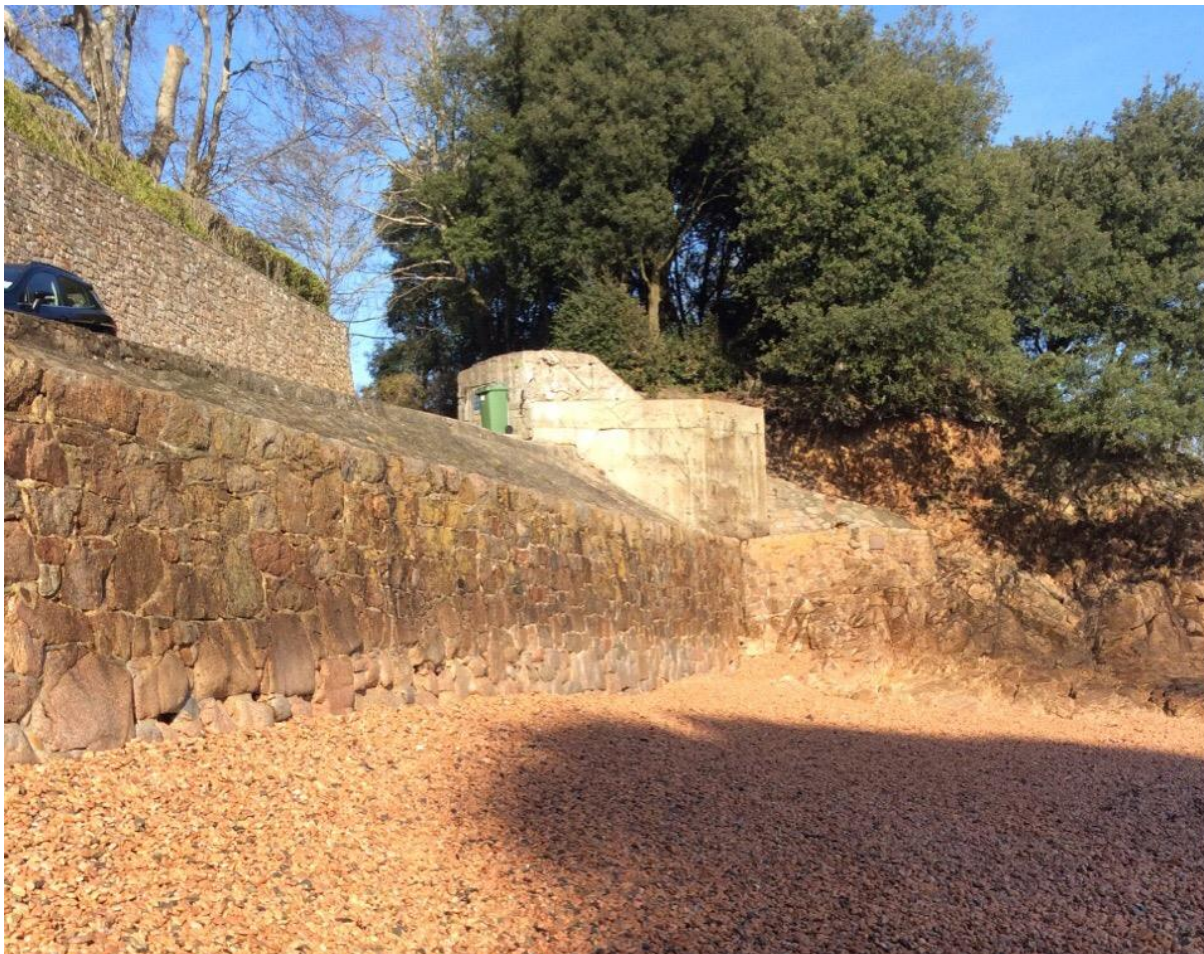
Figure 4-5: Vertical masonry wall at Belcroute Bay (CMU 1.2)
