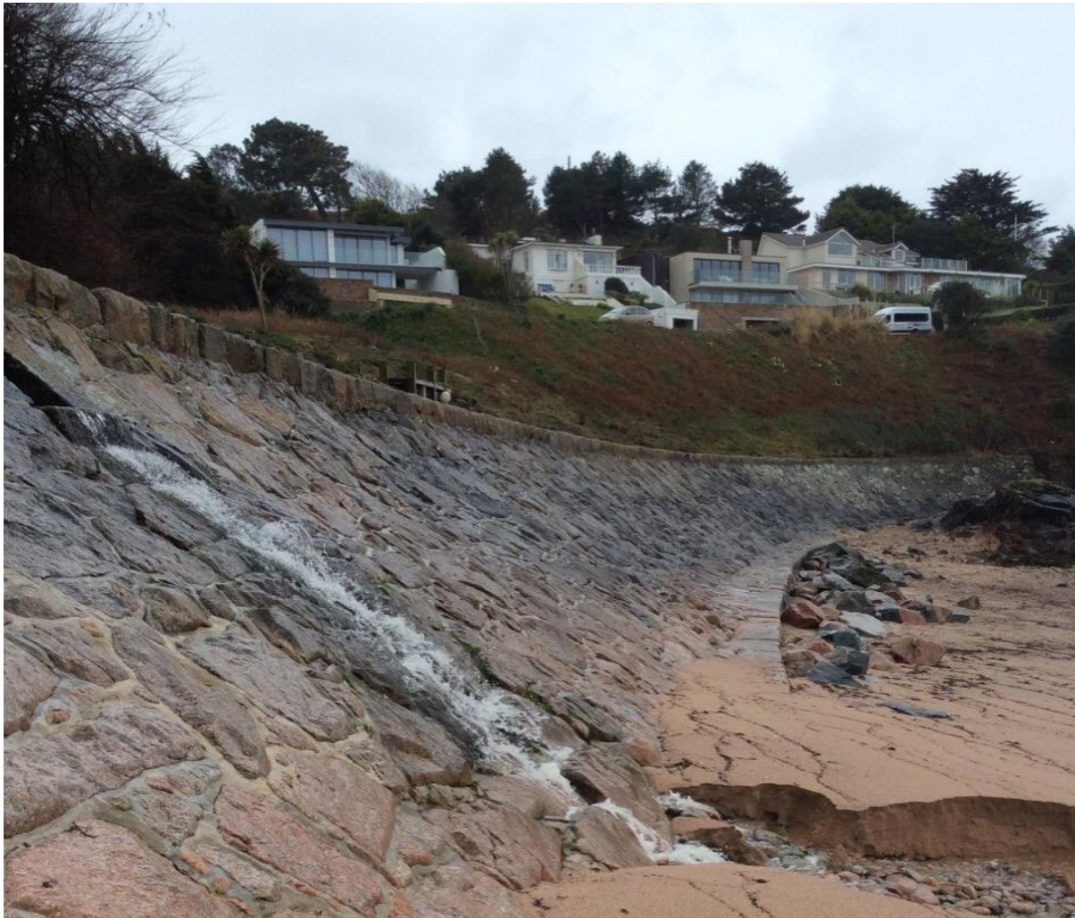
Figure 8-6: Coastal defences at Petit Port (CMU 5.2)
