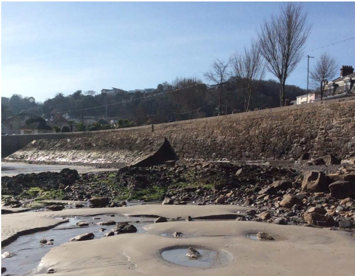
Figure 4-14: Sloping masonry wall at St Aubin's Bay (CMU 1.5)
