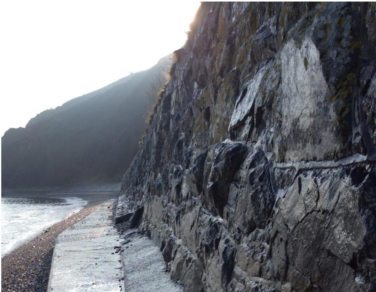
Figure 7-9: Coastal defences at Bouley Bay (CMU 4.4)
