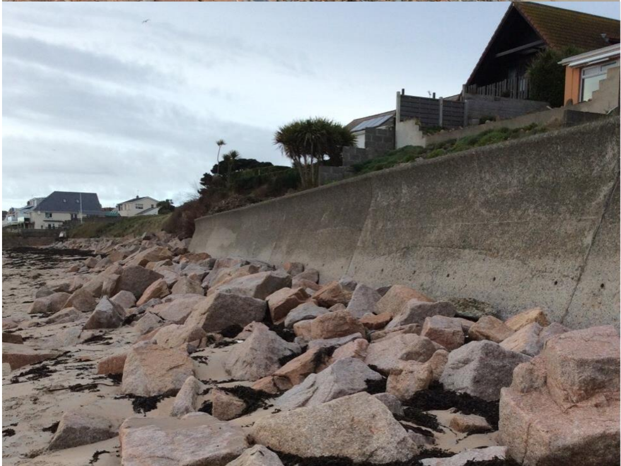
Figure 4-24: Existing defences at Le Hocq / Pontac (CMU 1.10)
