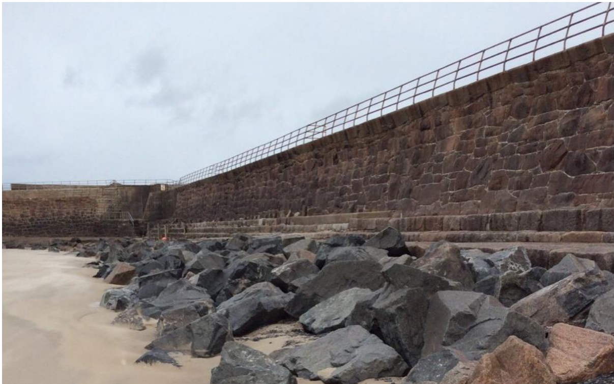
Figure 8-4: Coastal defences along St Ouen's Bay (CMU 5.1)
