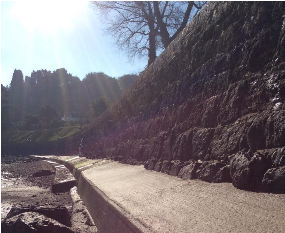
Figure 6-7: Coastal defences at St Catherine’s Bay (CMU 3.3)
