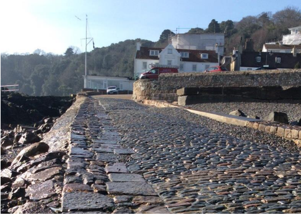
Figure 4-10: Existing coastal defences at St Aubin's Harbour (CMU 1.4)
