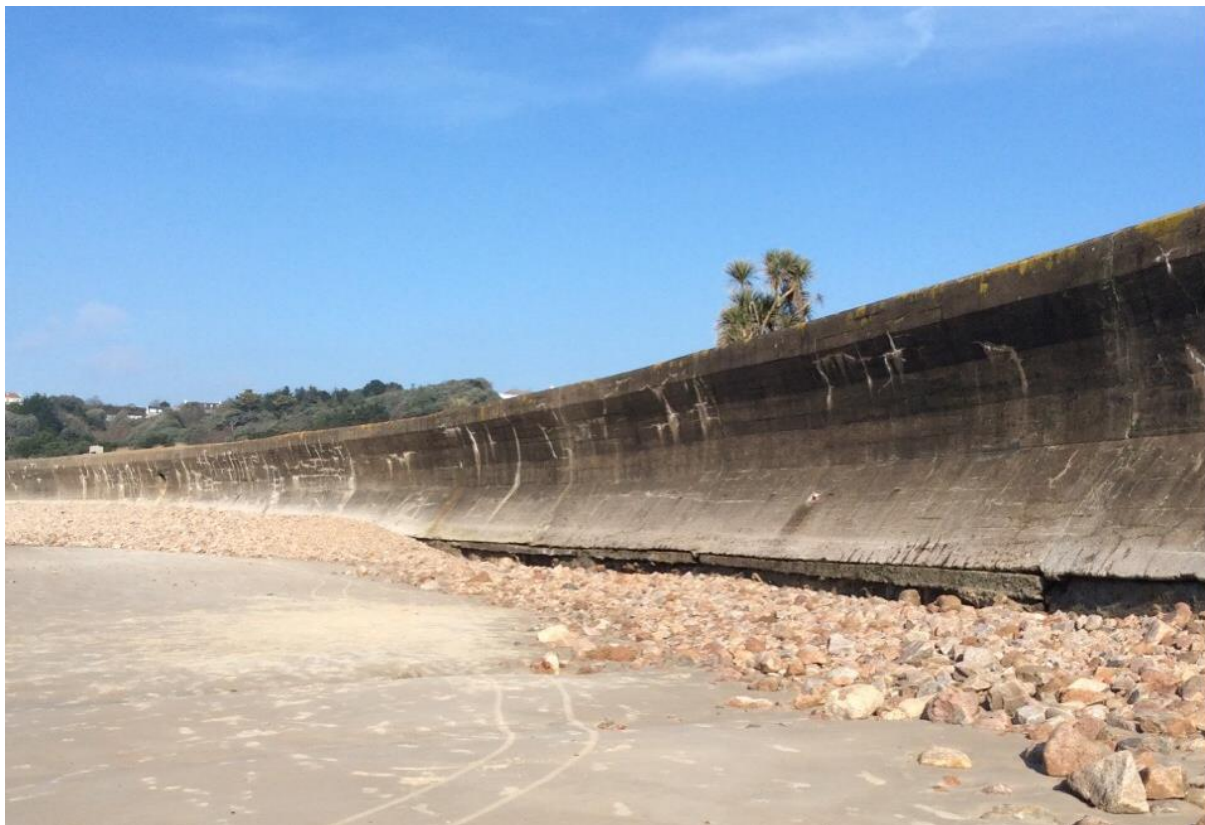
Figure 9-9: RC anti-tank wall at Ouaisne Bay (CMU 6.4)
