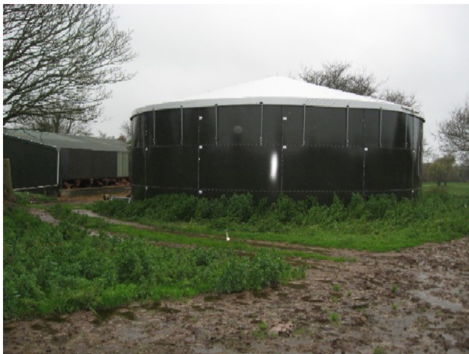
Figure 5 New slurry store to allow better use of slurry as a fertiliser.
