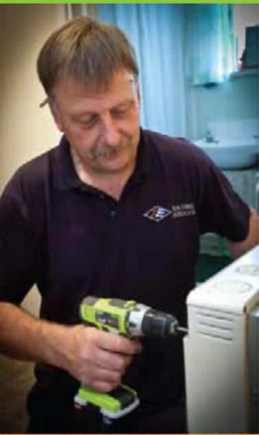
JEBS Electrical Engineer Derek Moon completes another fuel switch.
