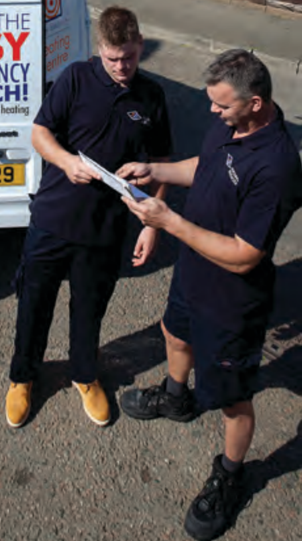
Danny Oberst and fellow JEBS Plumbing and Heating Engineer Doug Prentice discuss the replacement of hot water cylinders at Clos Gosset, part of the States Housing Fuel Switch Project.
