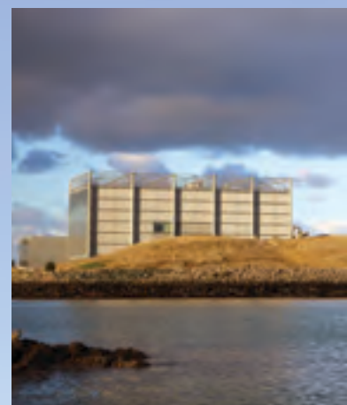
Energy from Waste (EfW) plant comes on line in Q1 2011.
