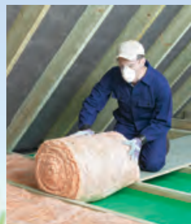
Installation of loft insulation is part of the Energy Efficiency Programme.
