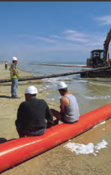
Laying of Normandie 2 from Saint Remy des Landes.
