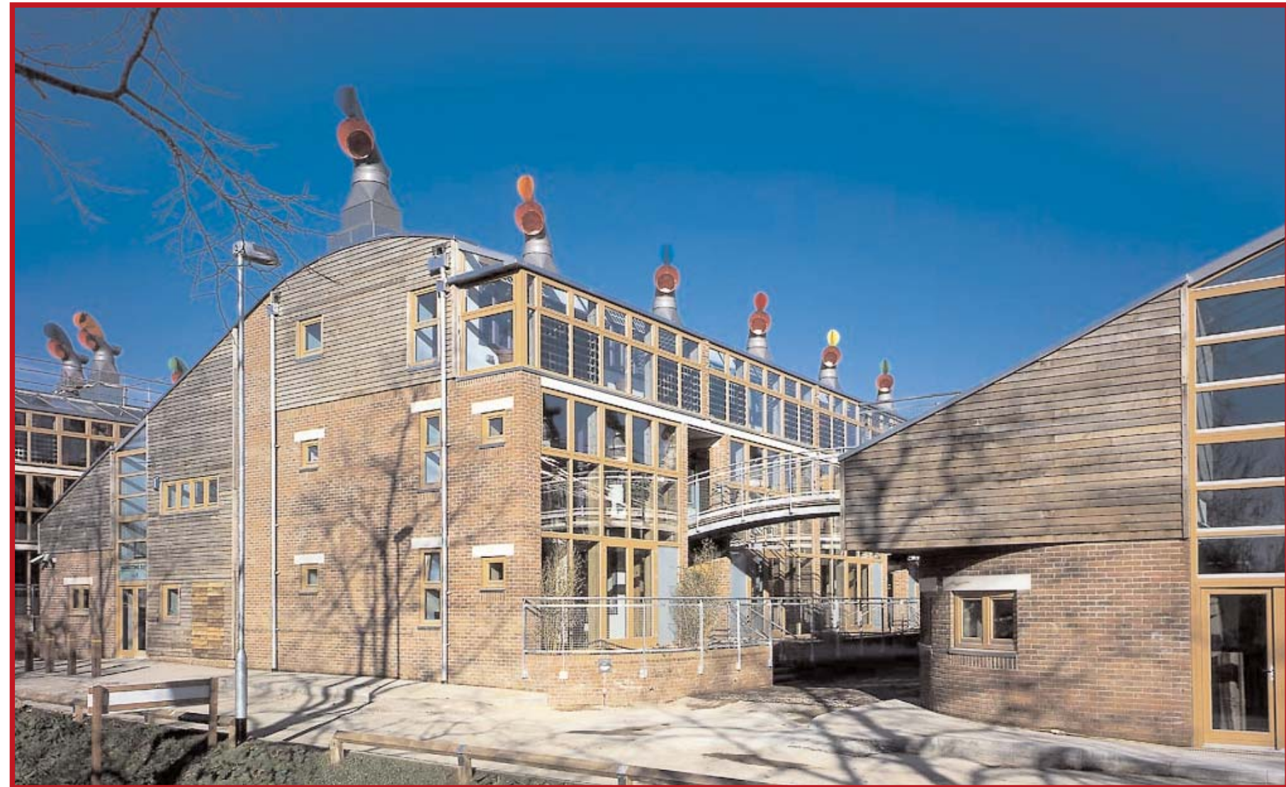
Above The gable end treatment of BedZED introduces a new urban typology using local traditional materials.
