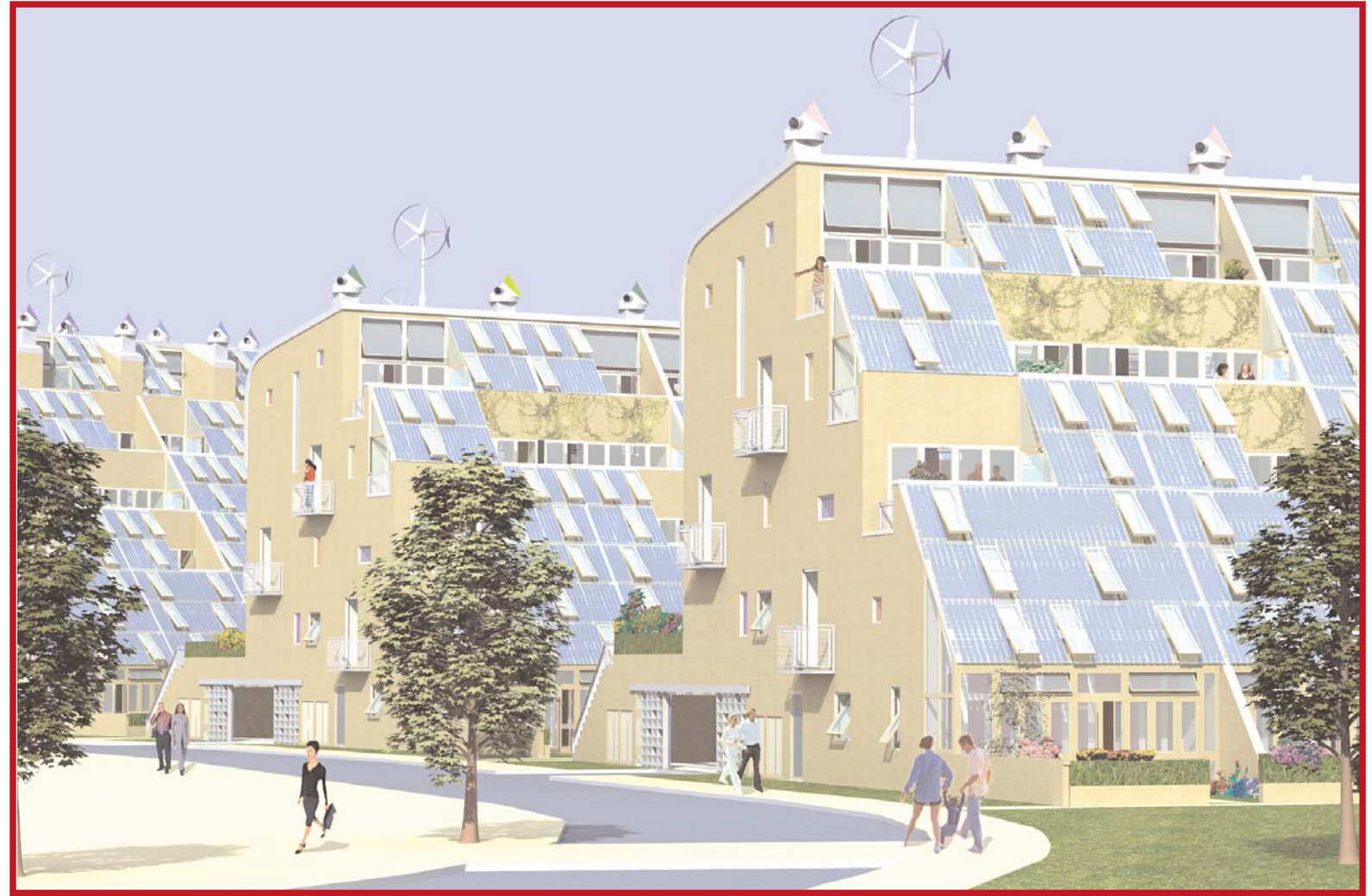
Above: Showing conservatories on South side, with building integrated PVs and some opening lights.
