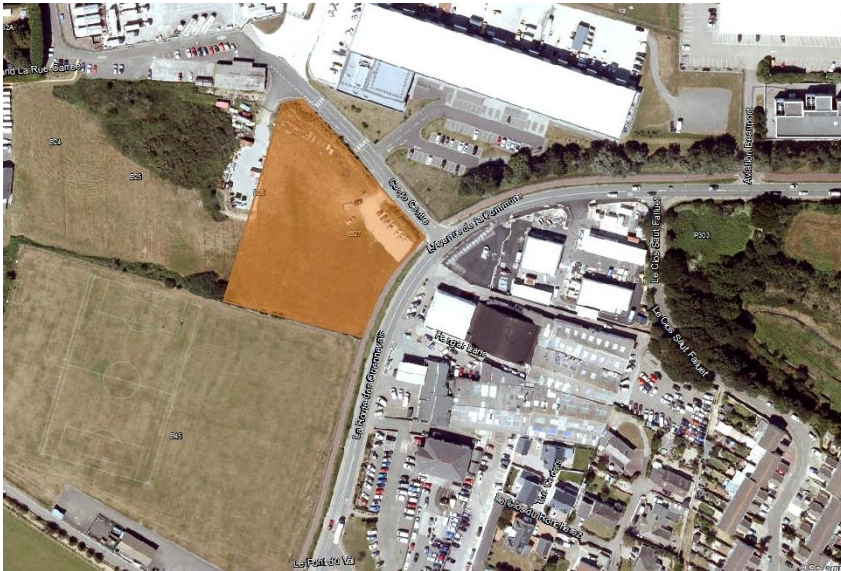
B26 and B27 La Route des Quennevais, St Brelade
