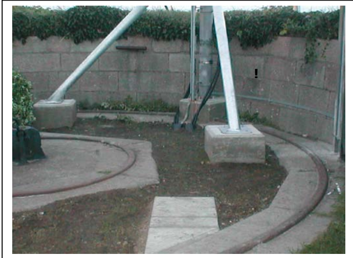
Communication mast installation Signal Station, 2006
