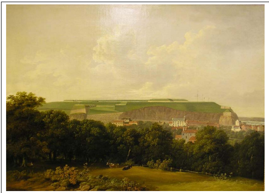
View of Fort Regent from the Northeast, Tobias Young c 1815-24 Courtesy of the Jersey Heritage Trust
