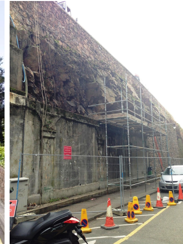
Current Stabilisation Work
