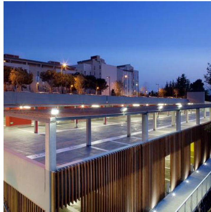
Example of permeable flanks and well lit upper surfaces
