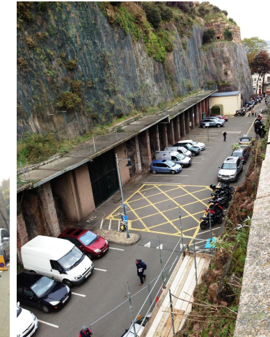
Cavern Access & JEC Substation
