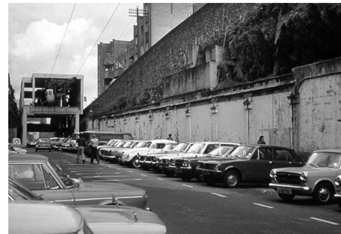
1973 with cable car & historic pillar mouldings
