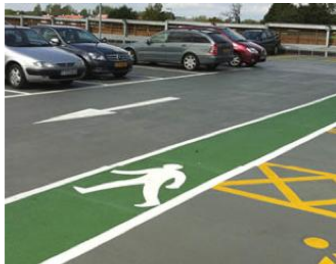
Coloured deck finishes helping designate areas
