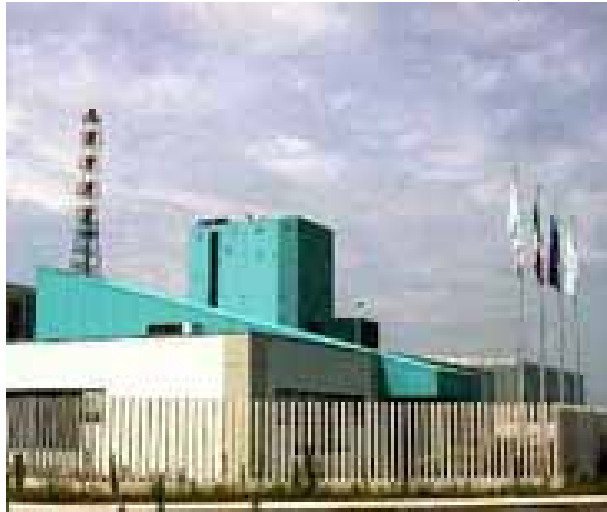
Picture of Lomellina RDF-fired plant, Italy (from FW Website)
