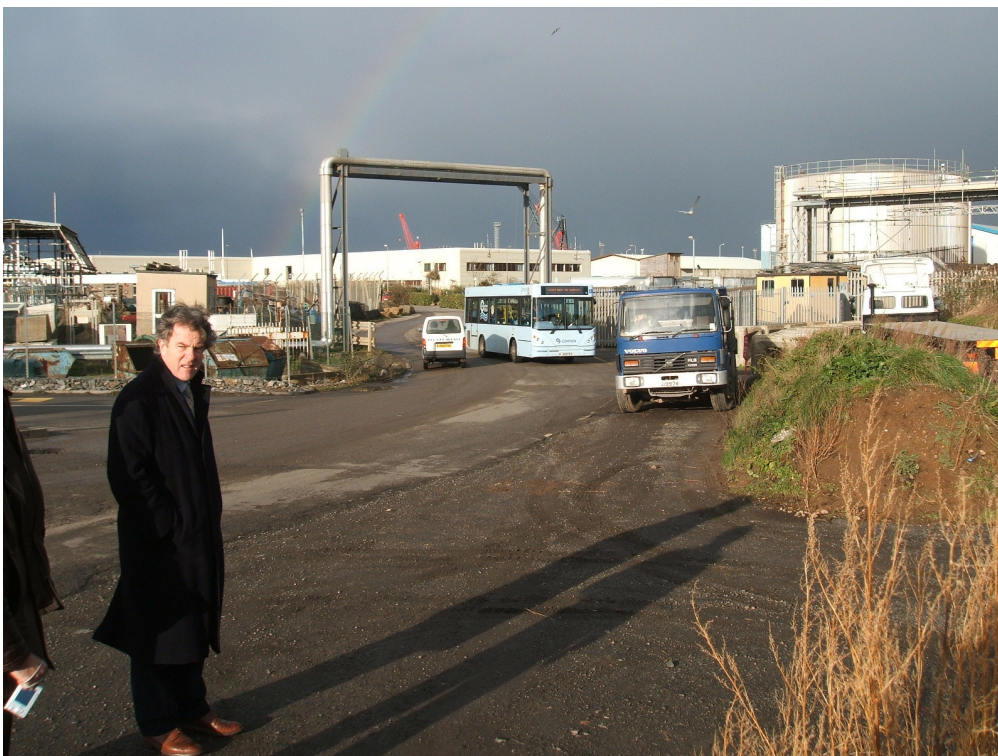
Fig 2 Pipe Bridge at the entrance to site.
