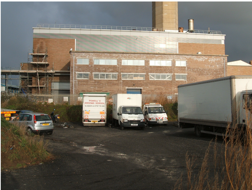
Fig 4 View on south elevation of La Collette Power Station
