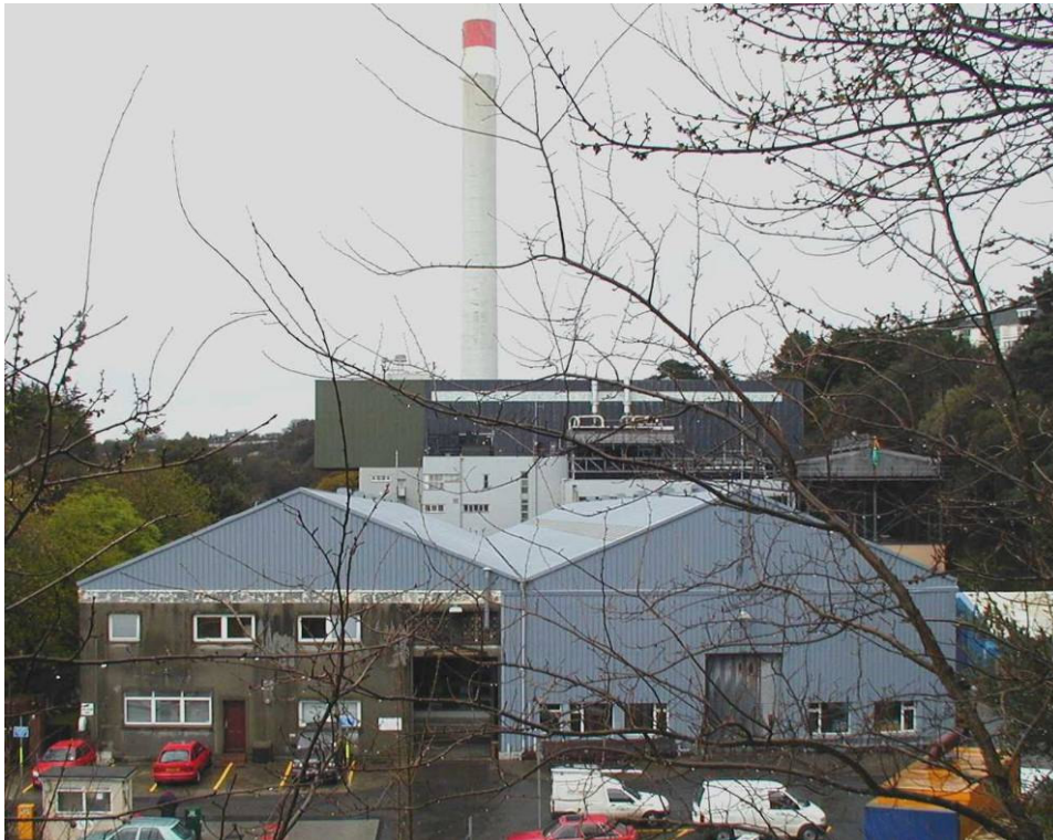
Existing Incinerator at Bellozanne
