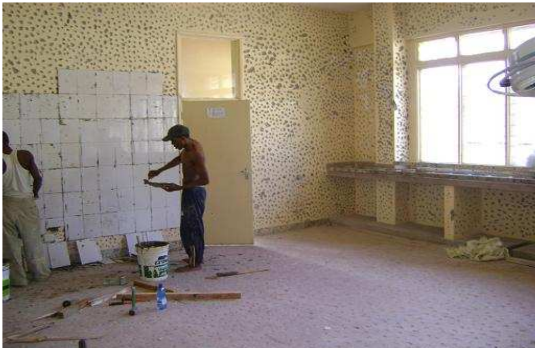
St Clements Church Operating theatre restoration, Kenya
