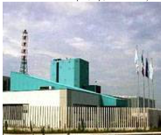
Picture of Lomellina RDF-fired plant, Italy (from FW Website)
