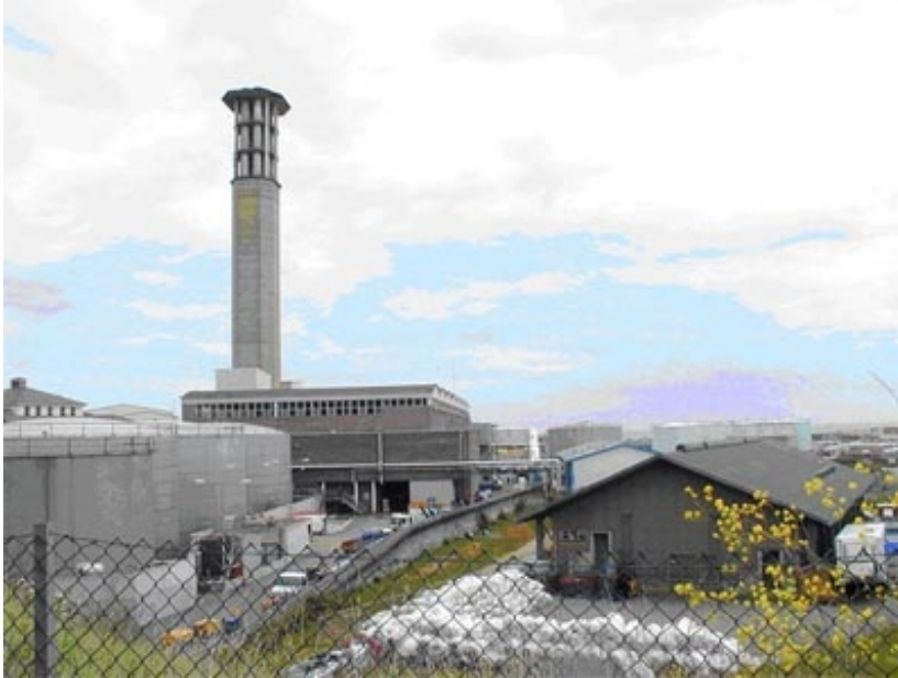
Photograph 2: The Jersey Electricity Company power station.
