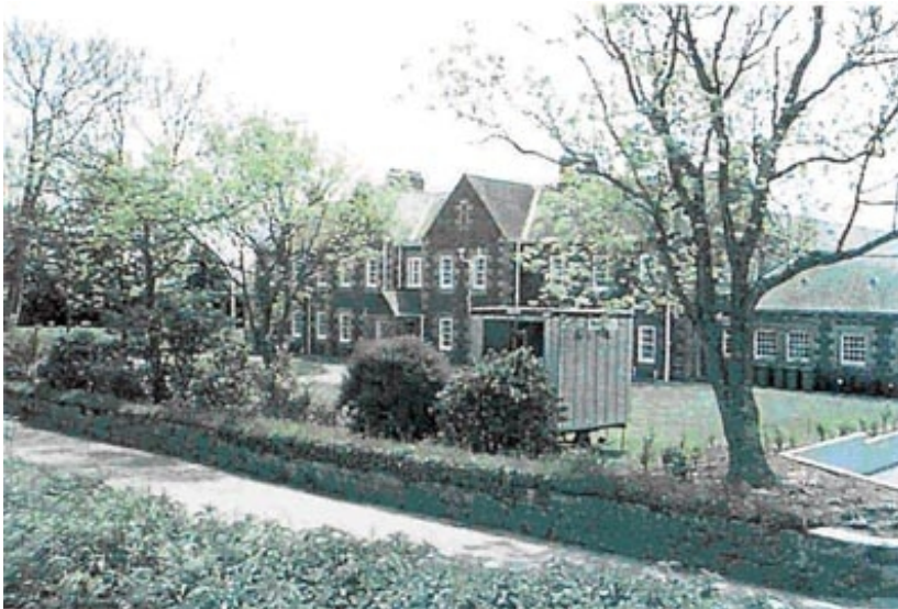
Photograph 1: The air pollution monitoring equipment housing is shown below.
