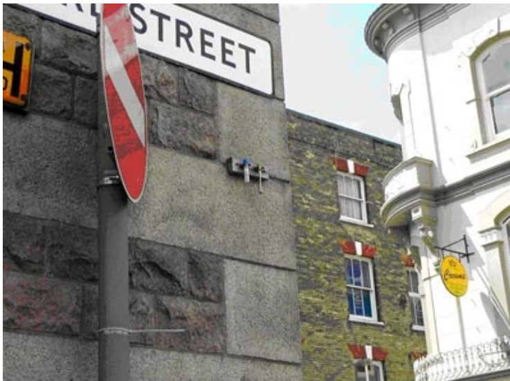
Photograph 4: Diffusion tubes placed on the building façade on the corner of Beresford Street, St Helier
