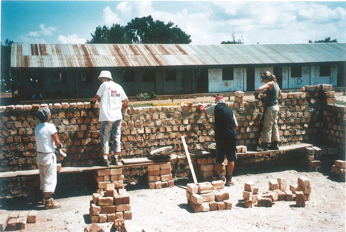
The library under construction, with team and 'helpers' below
