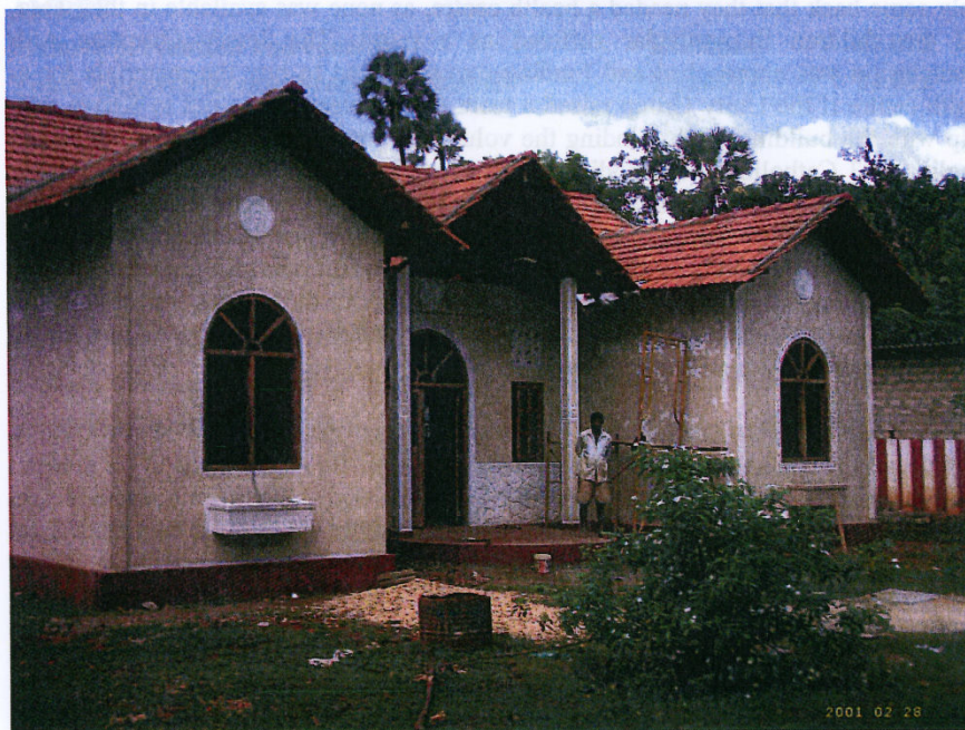
Newly Constructed Orphanage, Sri Lanka Island Friends Together
