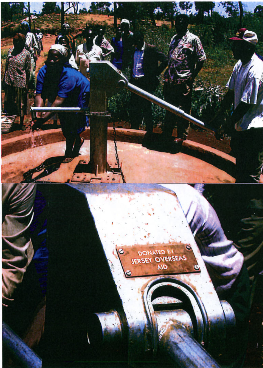
Newly installed well at Kakelo, Kenya Good News Trust
