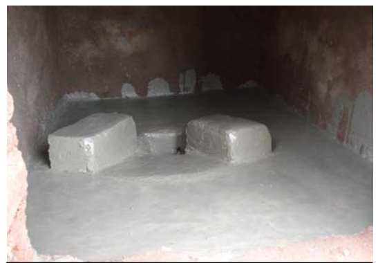
Close up of a latrine under construction
